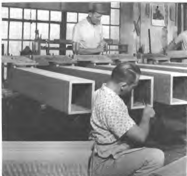
A section of the wood pipe shop.
