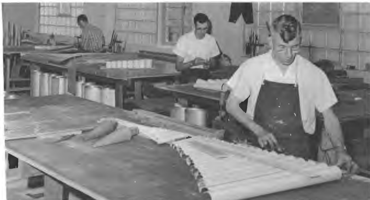
A view of a portion of the metal pipe shop.
