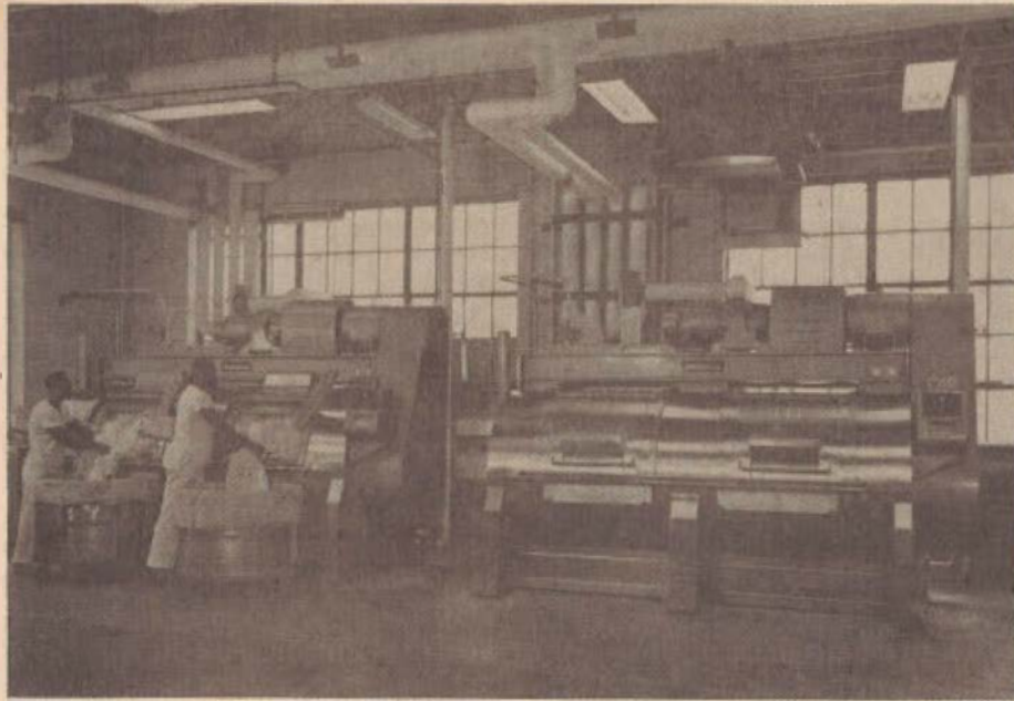
These are the kind of washers which will be installed in the new ABH laundry when it is completed. Each one will wash 600 pounds of clothes at a time.
