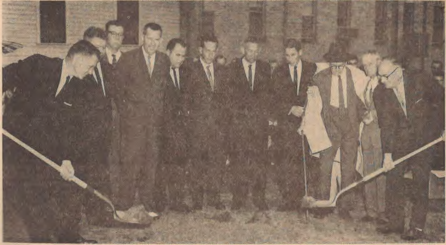
GROUND BREAKING —At Bluff Avenue Church, Ft. Smith, Easter morning for a new sanctuary, first of four units in a 12-year, $250,000 building program.
