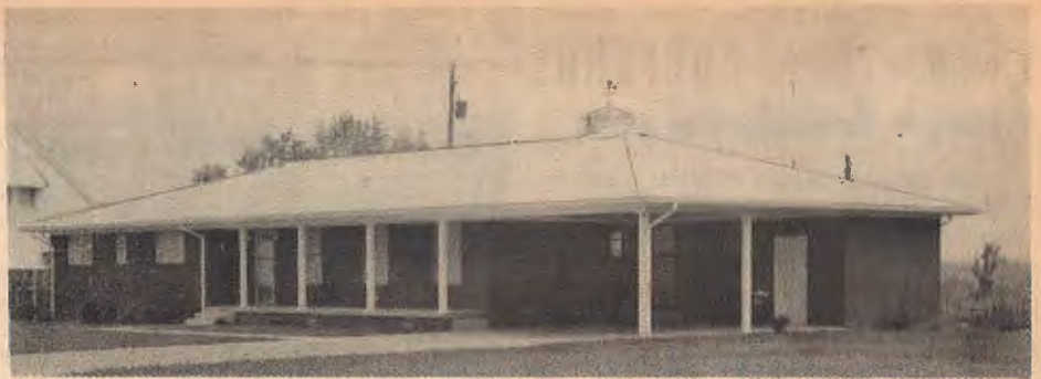
BATESVILLE WEST CHURCH PARSONAGE —The completion of a new four-bedroom parsonage by the church is listed as one of the numerous pluses in the church's year of accomplishment. Also listed is a record number of additions, 105, to the church. T. R. Coulter Jr. is pastor.
