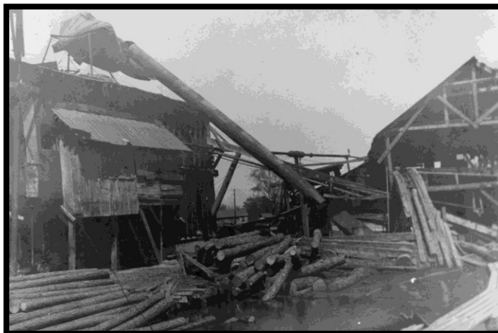
The Thomas Mill at Curtis suffered damage from a tornado in 1950
