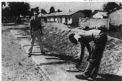
Missionary Brad Masbburn inspects pit toilet installation.
