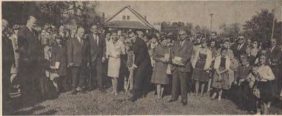
FT. SMITH FIRST GROUNDBREAKING —A colonial structure at the corner of 14th and E Streets in Ft. Smith will be built by First Church. Groundbreaking ceremonies were held Oct. 16. The sanctuary will seat 1,400. A suite of offices for church personnel will be housed in the new building, which will cost $730,500. Pastor Dan T. Cameron, above, turns the first shovelful of dirt. Completion is expected in one year.
