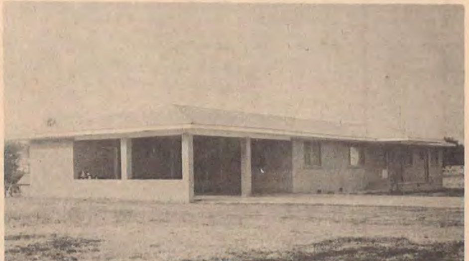
MONTICELLO—This $30,000 brick parsonage was recently completed here by Second Baptist Church and is now occupied by the church's pastor and family, the Bill H. Lewises. The home has four bedrooms, two bathrooms, a family room, kitchen with built-in fixtures, living room, dining room, two utility rooms, and a double carport. It is centrally air conditioned and heated.—ABN Photo
