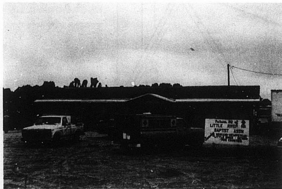
Little River Association, comprised of 26 churches, recently completed construction of an office/resource center as a result of the cooperative efforts of the Arkansas Baptist Church In A Day Builders and the Little River Association Volunteers. Ken Conway of Ashdown served as building committee chairman. Charles Cunningham of Ashdown was architect and James Cannon, associational director of missions, coordinated the project. Meals were supplied by area Southern Baptist churches and served by Bernice Box of Ashdown, director of Little River Association Woman's Missionary Union, assisted by Wilma Cannon of Lockesburg and Gay Nell Baskin of Oak Grove.
