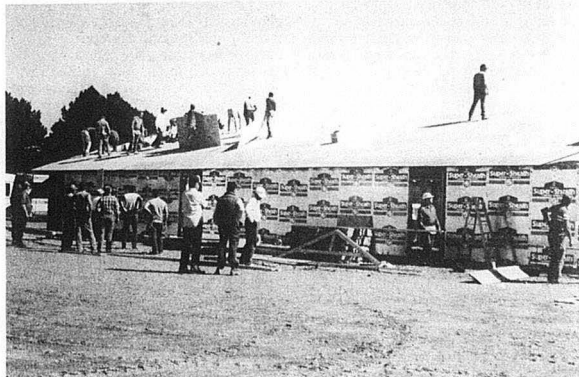
Teams of Baptist Men work to complete Crestview construction.
