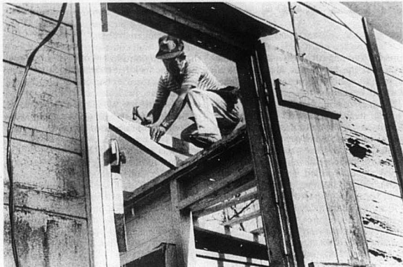
Georgia layman Richard Parker repairs a roof in Guadeloupe.
