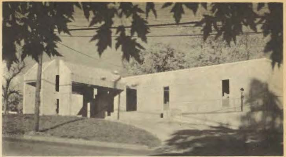
This is the new pre-school building of First Church, Siloam Springs. The building is 49 feet by 98 feet and houses all pre-school children. It also provides space for a kindergarten, which the church operates, and is to be the home of a day-care center which is now being planned, Bill Bruster, pastor, reports.
