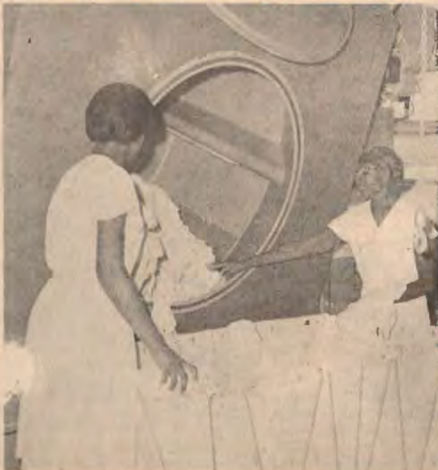
At left, two laundry employees unload the big drier which dries up to 250 pounds of clothes every 15 minutes. At left the new ironer carries linens through at the rate of 125 feet per minute.
