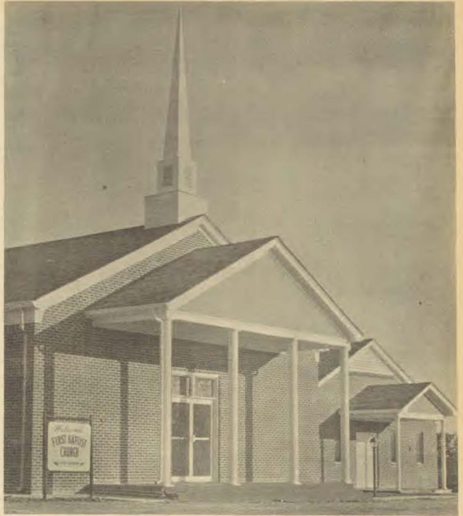
The newly remodeled building
