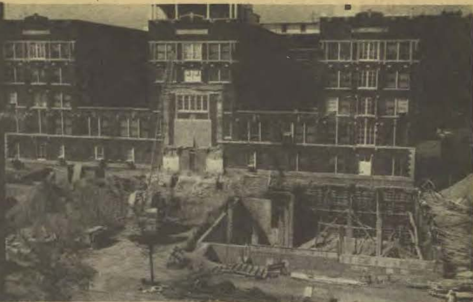
This view of the front of Arkansas Baptist Hospital shows progress of construction of the new $1,500,000 addition. This shot was made Sept. 15, just two months and three days after ground was first broken for the new building.
