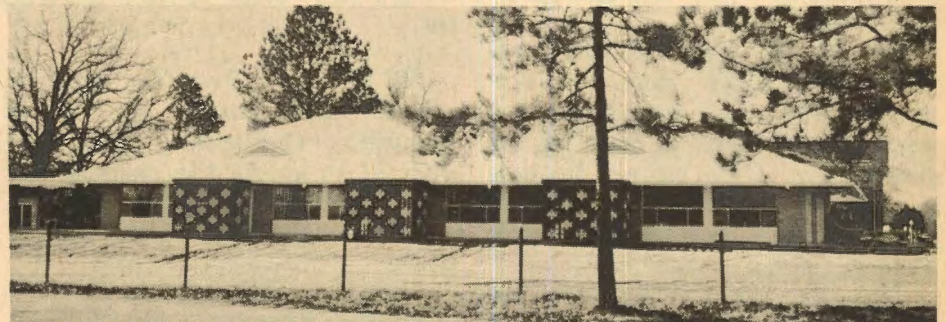
FIRST Church Prescott, dedicated its new educational building Feb. 14 at the Morning Worship service. The new building will accommodate the Nursery, Primaries, Beginners and Young Peoples' departments. One Adult Department will be in the building. A kitchen and dining area are included. Open house followed the dedication.
