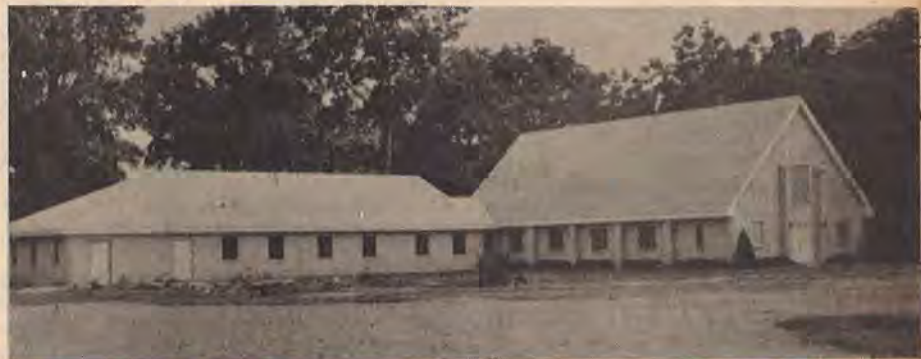
ARKANSAS CITY Church recently dedicated a new educational building (left), with Dr. S. A. Whitlow, executive secretary of the State Convention, speaker. The 54-by-87-foot building houses nursery through young peoples departments, with rest rooms, kitchen and air-conditioning. Reese S. Howard is the pastor.
