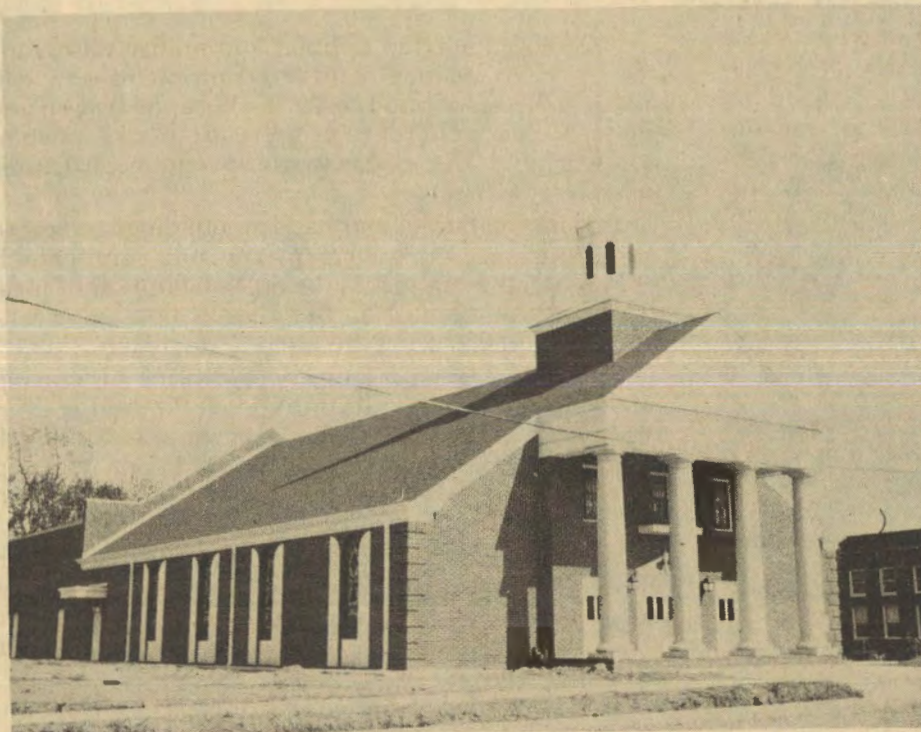
First, Booneville, has completed this auditorium-education complex.
