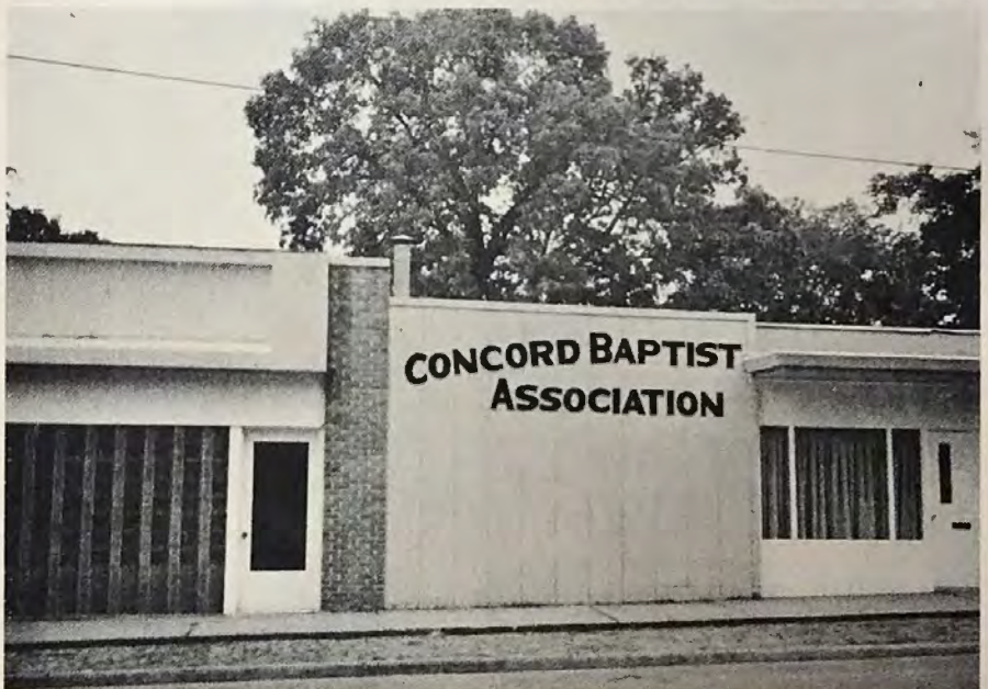
Concord Association bought this building in 1971 and renovated it for use as the Associational office.
