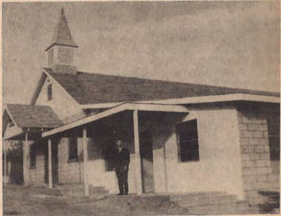
SECOND CHURCH, Van Buren, dedicated its new educational building (above) Feb. 17. The modern 13-room building, constructed through the labor of the church membership and the financial assistance of the state Mission Department, was presented to the congregation by Clyde Raymond Smith, deacon. Participating in the dedicatory service were Rev. George Lonsbury, former pastor, Rev. Paul E. Wilhelm, Clear Creek Association missionary, and Rev. Robert Morrison, present pastor. The church was organized in 1958.
