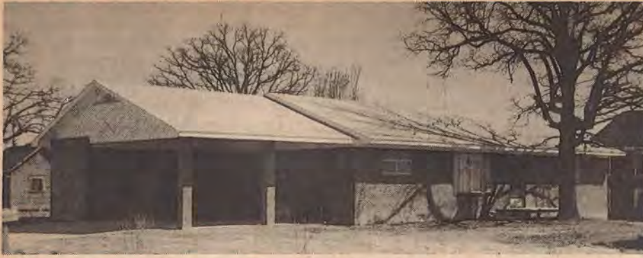
DALLAS AVENUE parsonage: Open house for the new, three-bedroom home for the pastor of Dallas Avenue Church, Mena, was held March 31. The brick residence has 1,928 square feet of floor space, including a study. Draperies for the home were provided through gifts from the women of the church. Rev. W. T. Byrum is pastor.
