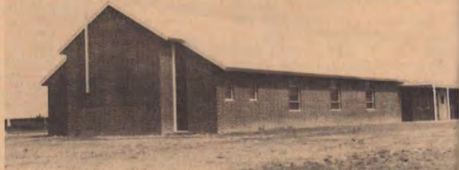
NEW BUILDING recently dedicated by Elmdale Church, Springdale, contains an interim sanctuary and departments for nursery through Intermediate classes.
