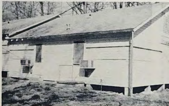
Twenty Four Air Conditioned Family Units
