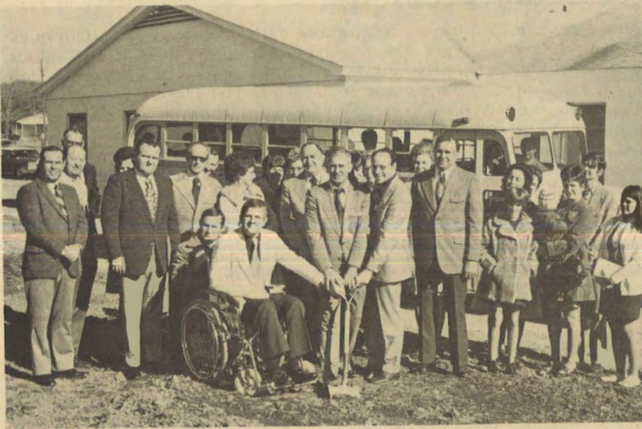
Ridgeview Church, Fayetteville, held a groundbreaking service recently for the construction of a new building to accommodate its growing membership. The church received 75 new members through baptism last year. Pastor Doyle Wesson declares "Our growth all began with one bus which is now expanded to six as well as a children's church." Pictured are the members of the building and finance committee and some of the members of the church. In the center, holding the shovel, is pastor Wesson. To his right is Assistant Pastor Jack Taylor.
