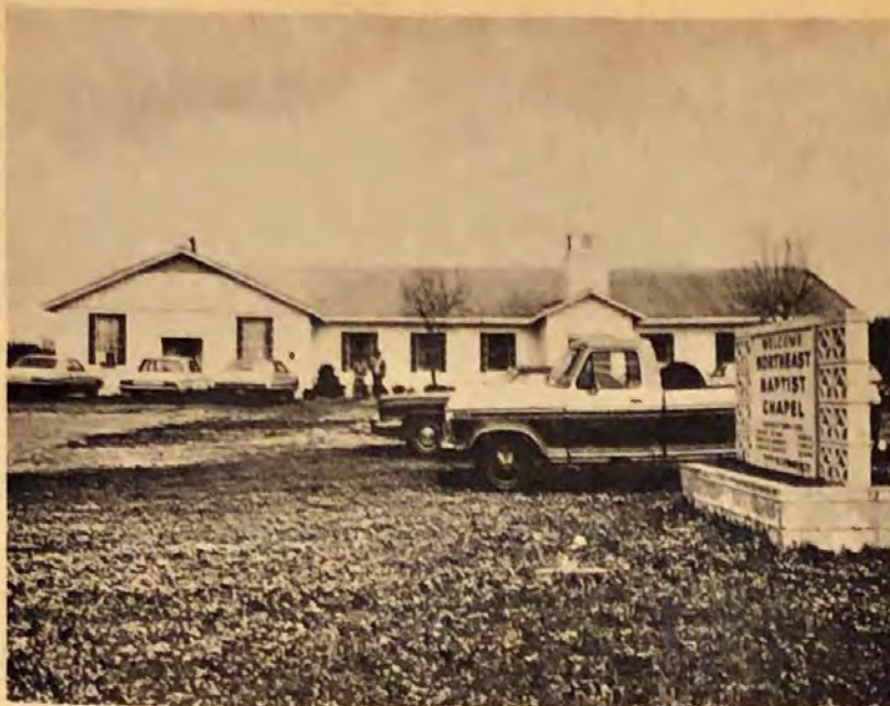
The chapel met, and the new church meets in this building.
