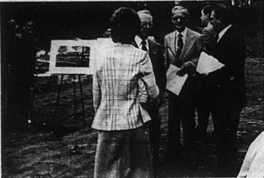
Little Rock Baptist Medical System broke ground Nov. 11 for a retirement community, Parkway Village. The $40 million, 600-unit community, to be located in western Little Rock, will be built in three phases and is expected to be completed within five years. Don Moore, Executive Secretary of Arkansas Baptist State Convention, and W. O. Vaught, pastor of Immanuel Church in Little Rock, participated in the service. Moore (far right), speaker for the occasion, visits here with some of the groundbreaking guests, including R. H. Dorris (third from left), a former president of the Baptist Medical System Board of Directors.
