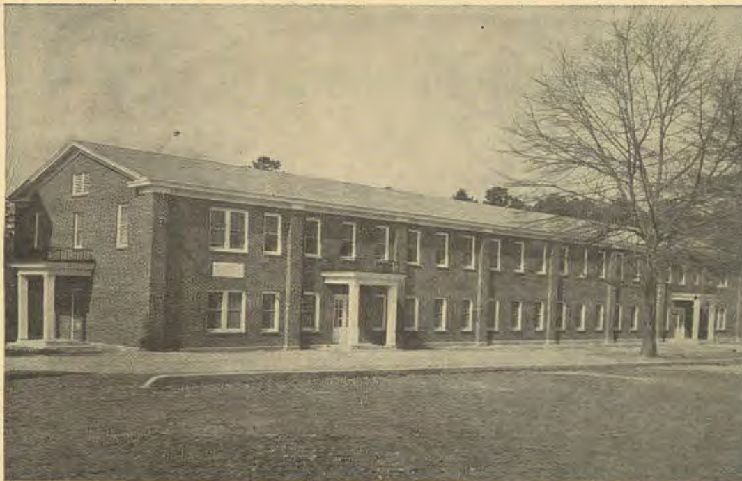
TERRAL-MOORE HALL, GIRLS' DORMITORY A CAMPAIGN BUILDING COMPLETED
