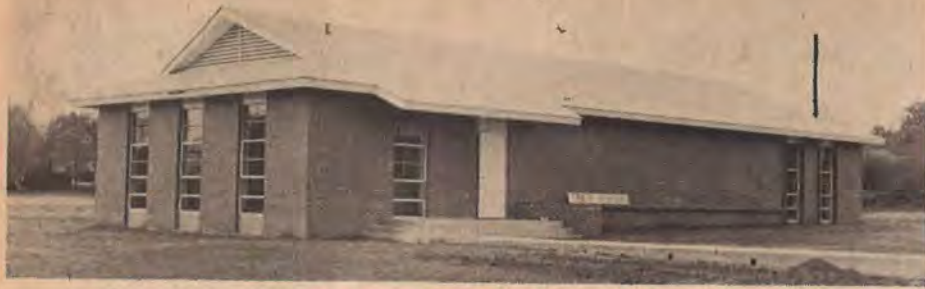
NEW CHURCH —Trinity Church at Searcy, dedicated recently, is the first unit of a four unit building planned. The new building seats 100 in a temporary auditorium and has nine class rooms and complete kitchen. Rev. David M. Stevens is pastor.
