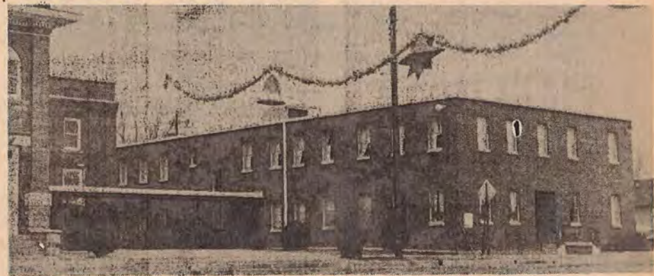
EDUCATIONAL Building of First Church, Booneville, was dedicated recently and the note burned. Principal speaker was Rev. D. B. Bledsoe, former pastor. The present pastor is Rev. Norman E. Lerch.
