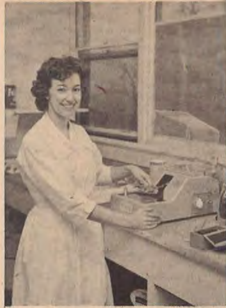
Technician Joyce Moore shows how the microtone blade is put into the new automatic knife sharpener.
