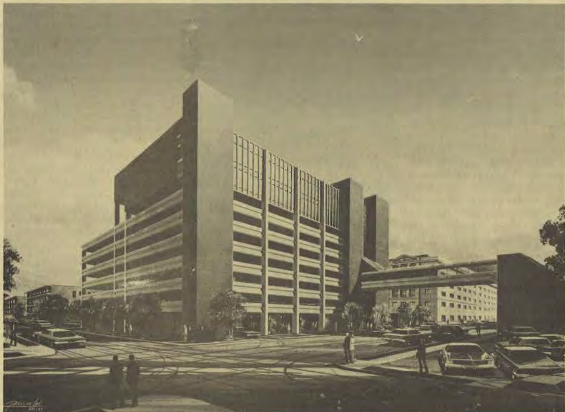
View from the southeast
