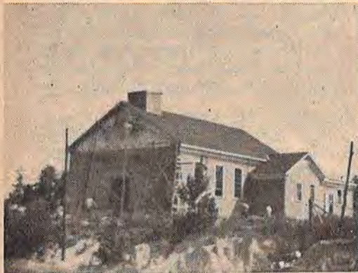
New church building at Camden Ordinance plant. Church was organized in June. The Mission Department purchased the ground and First Church, Camden, sponsored the services and construction.
