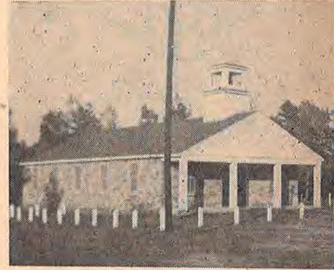
Bethel Church, Red River Association. The Mission Department gave financial assistance on the building.
