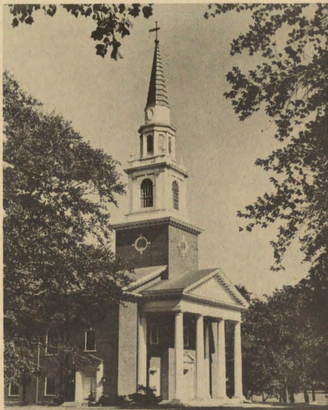
ALUMNI MEMORIAL CHAPEL, center of worship at The Southern Baptist Theological Seminary, 2825 Lexington Road, Louisville, Kentucky, was built in 1950, with gifts from alumni and friends. Styled in modified Georgian architecture, the Chapel seats more than 1,600. Its 113-rank pipe organ is the largest in the South.
