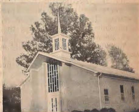
LEXA Church dedicated its new auditorium in special services recently. The new building has a seating capacity of 250 and is centrally heated and air conditioned. Glen Hicks is pastor.
