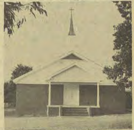
Holland Church's building was paid for as it was built.
