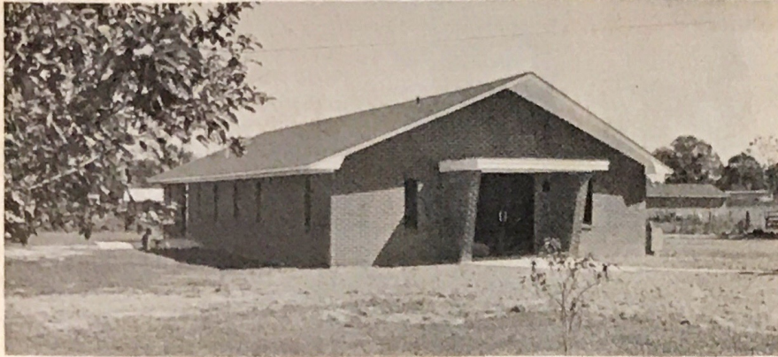
Donated labor helped the members of the Ward church build and furnish this building for $33,500. (ABN photo)
