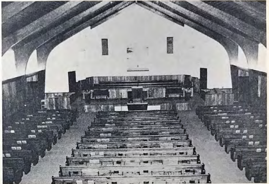
New auditorium for Eagle Heights Church, Harrison.
