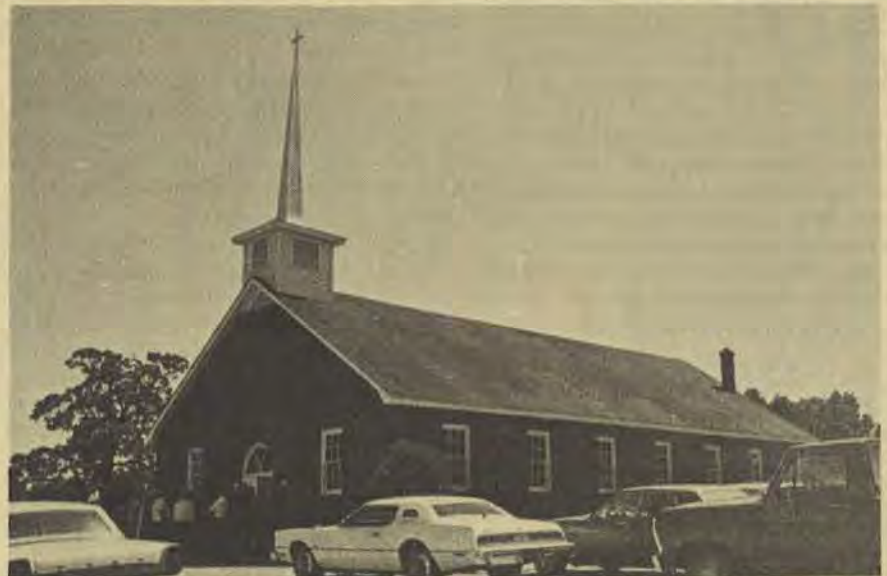
One of the things being celebrated by the Pollard Church was the improvement of their building.
