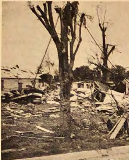
Power lines drape trees which have been nearly shorn of their branches.
