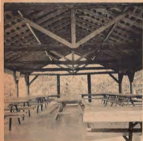
New Dining Hall—Under Construction
