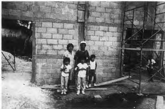
Pastor Jorge Cerritos and his family stand inside the church under construction.
