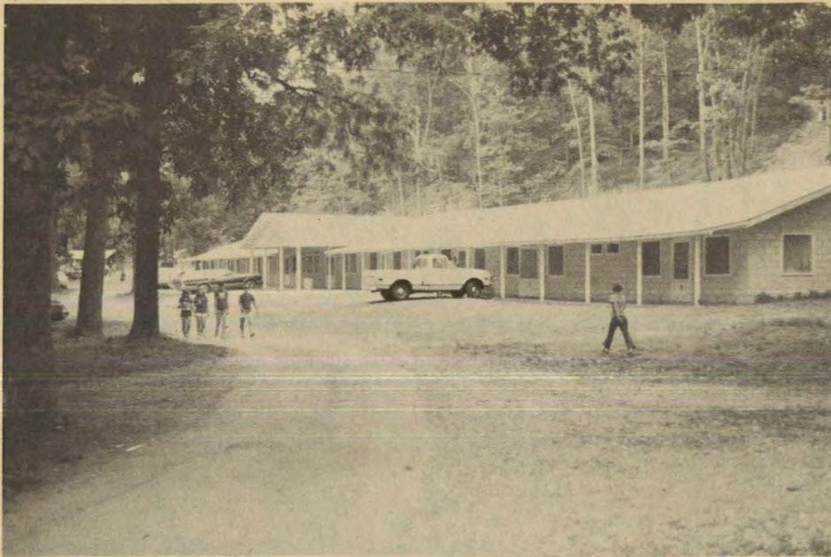
This is the Siloam Springs assembly facility which is winterized for up to 100 campers.
