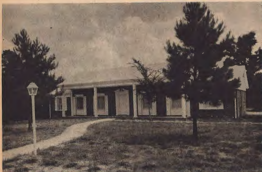
HOPE PASTORIUM —Completed this year is the brick veneer pastorium of First Church, Hope, at a cost of $40,000. The home, occupied by Pastor Gerald W. Trussell and his family, contains a large living-dining area, den-kitchen area, a study, three bedrooms, two full baths, a double carport and patio. It is centrally heated and air conditioned.
