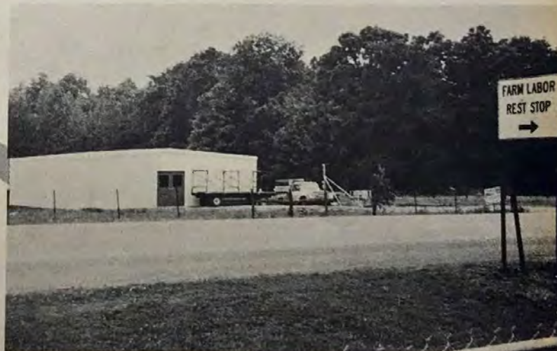
MIGRANT CENTER. (Below) As many as 60,000 migrant persons pass through the government rest stop at Hope each year. Arkansas Baptists now own a building across the road, with Robert Gross as full-time director, to provide a ministry to these people. Opened in May, the Center has already been visited by hundreds.
