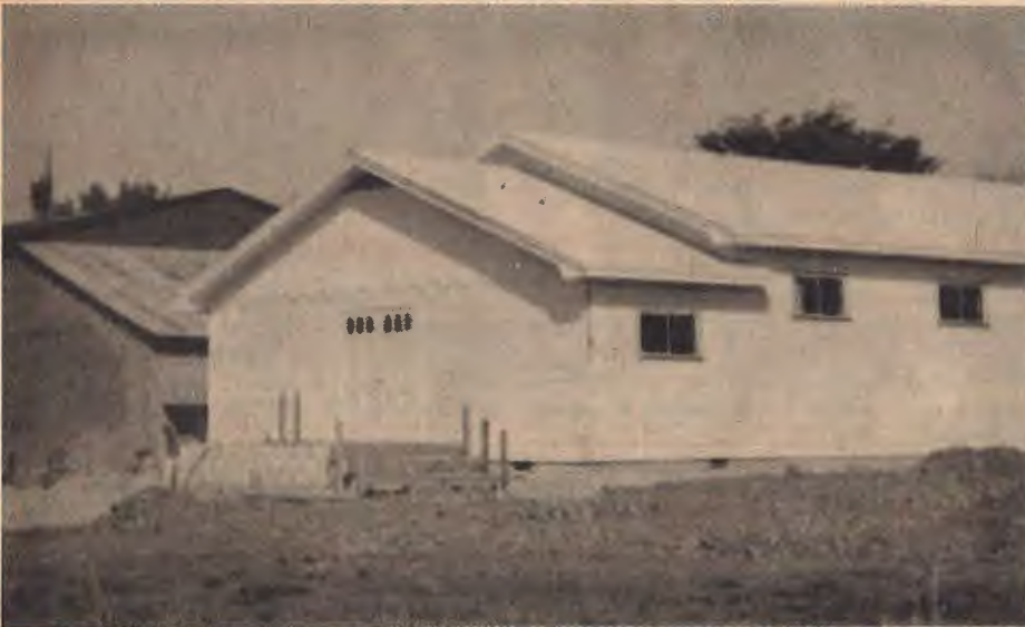
DEDICATED —Uniontown Church, north of Van Buren, dedicated a new 1800-square-foot church building Apr. 30. The frame building has an auditorium that will seat 200. Additional space is provided for four classrooms and a nursery. The hardwood-floored auditorium has indirect lighting, and the entire building has central heating. Edward Baker is pastor.
