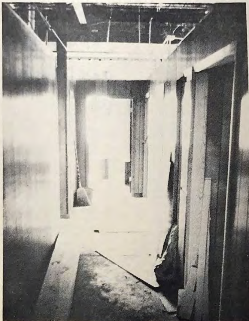
Interior renovation work on the administration building continues.
