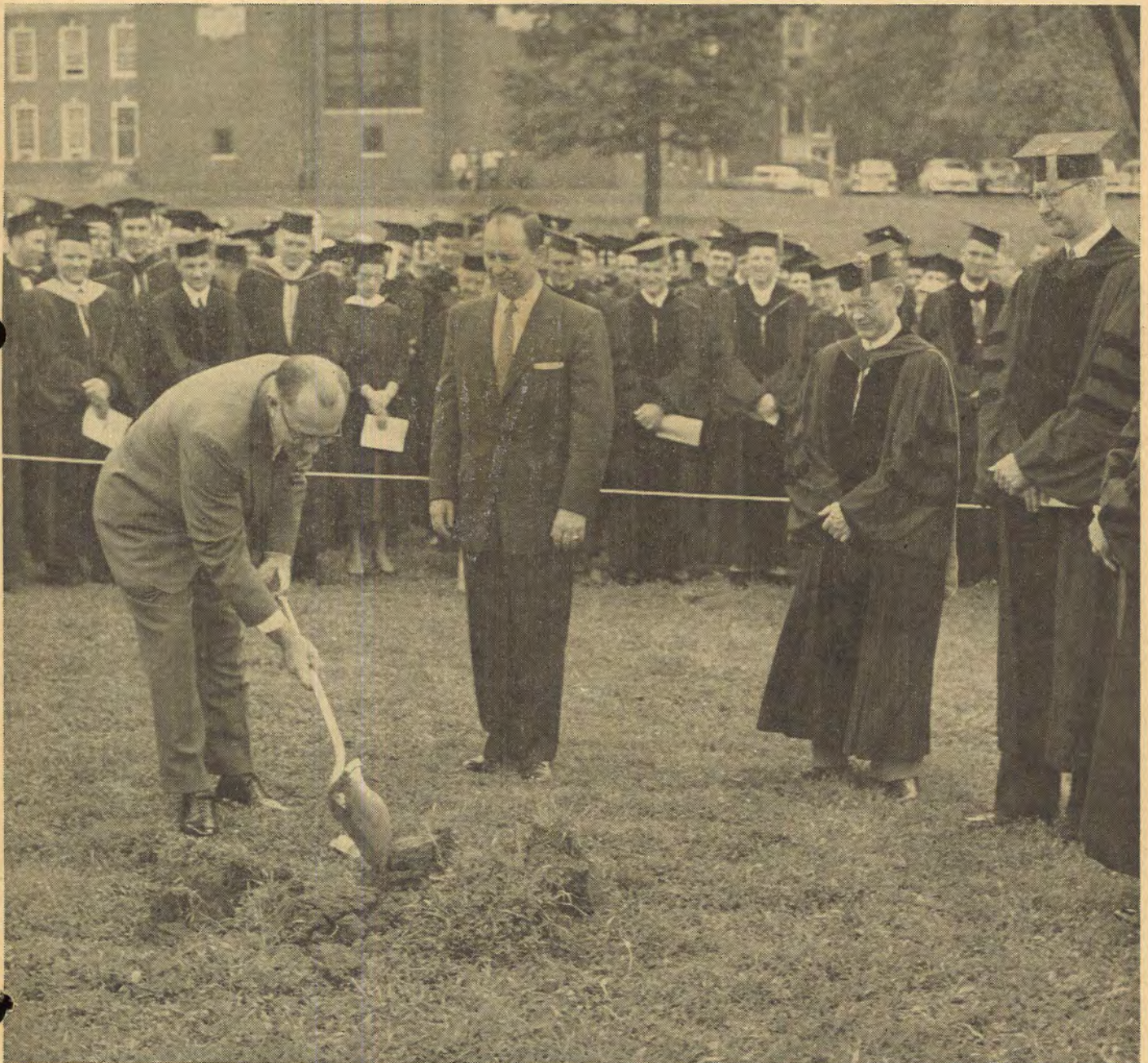
Groundbreaking at Southern
