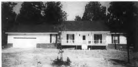
Owensville Church, located west of Benton on Highway 5, recently completed the construction of a parsonage in which pastor Larry D. White and his family are residing. The home was built on property adjacent to the church that was donated by church member Hugh Davis. Valued at $125,000, the parsonage was constructed at a cost of $67,000 by volunteers from Arkansas, Oklahoma, Missouri and Kansas.
