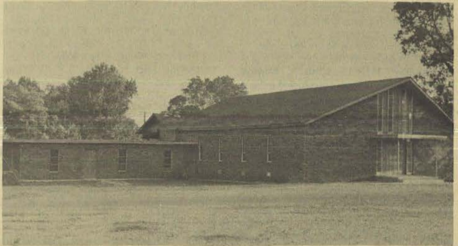
When the church built the education space at left, they also remodeled the sanctuary, changing its appearance on the outside by applying brick and adding stained glass for the foyer.
