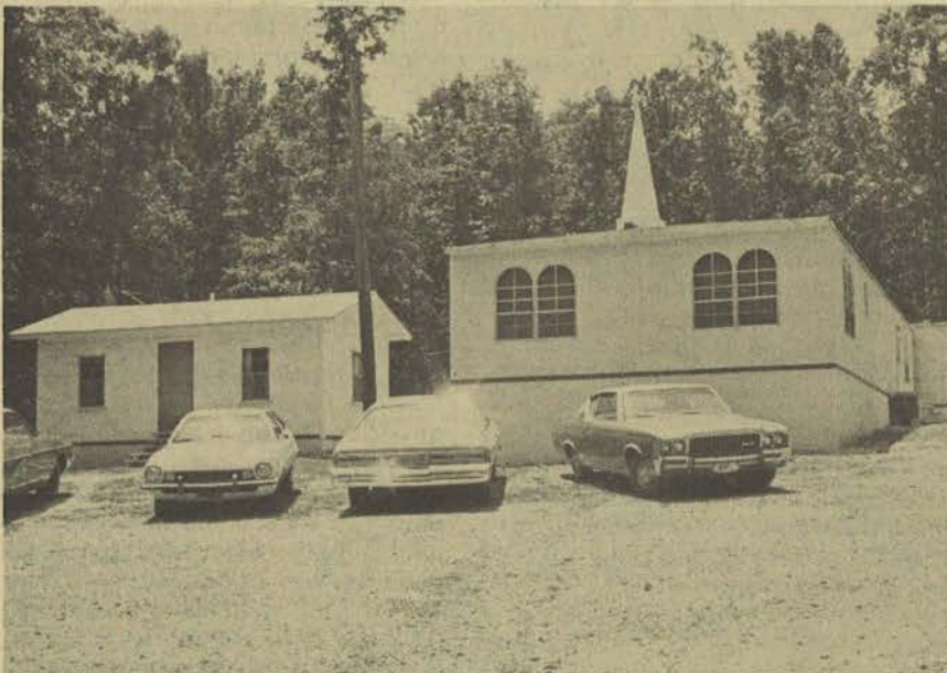
Hilldale Mission's prefab building provides them with 3,456 sq. ft. at a cost of just under $21,000. They dedicated the building Sunday, June 5. (ABN photo)
