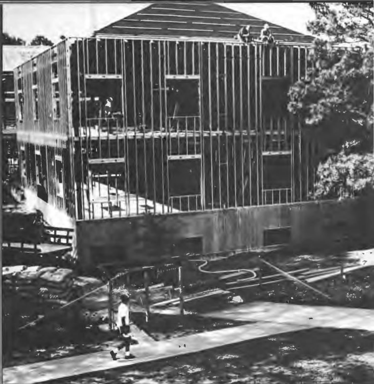
Going up. Workers from Pickens-Bond Construction build the frame to the new Riley-Hickingbotham Library. The facility was completed for student use in the fall.
