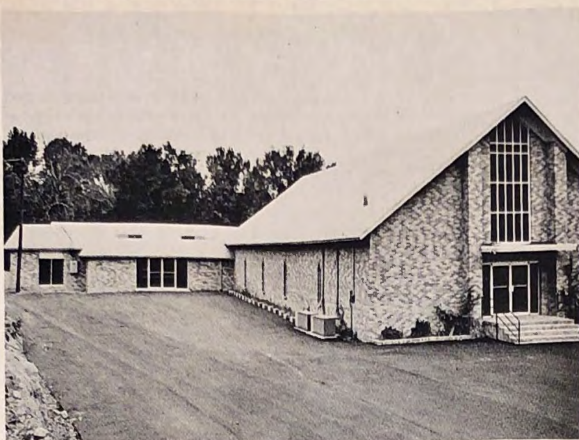
The educational addition is at the left of the auditorium.
